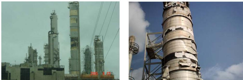
**Figure 95. Observed Hurricane Damage to Process Towers**
