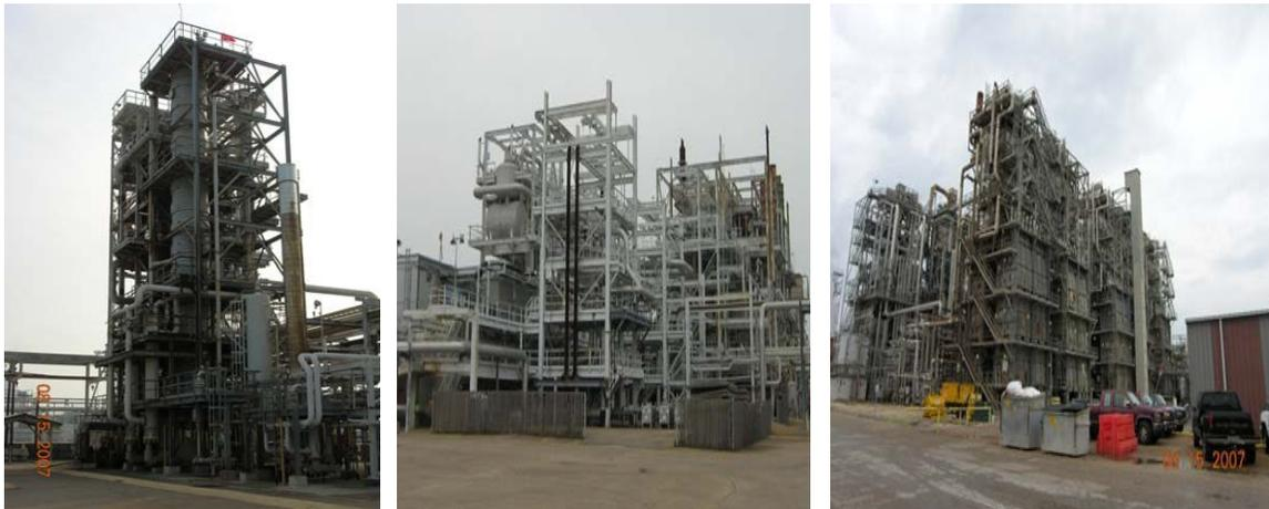
**Figure 91. Examples of Open-Frame Structures**
