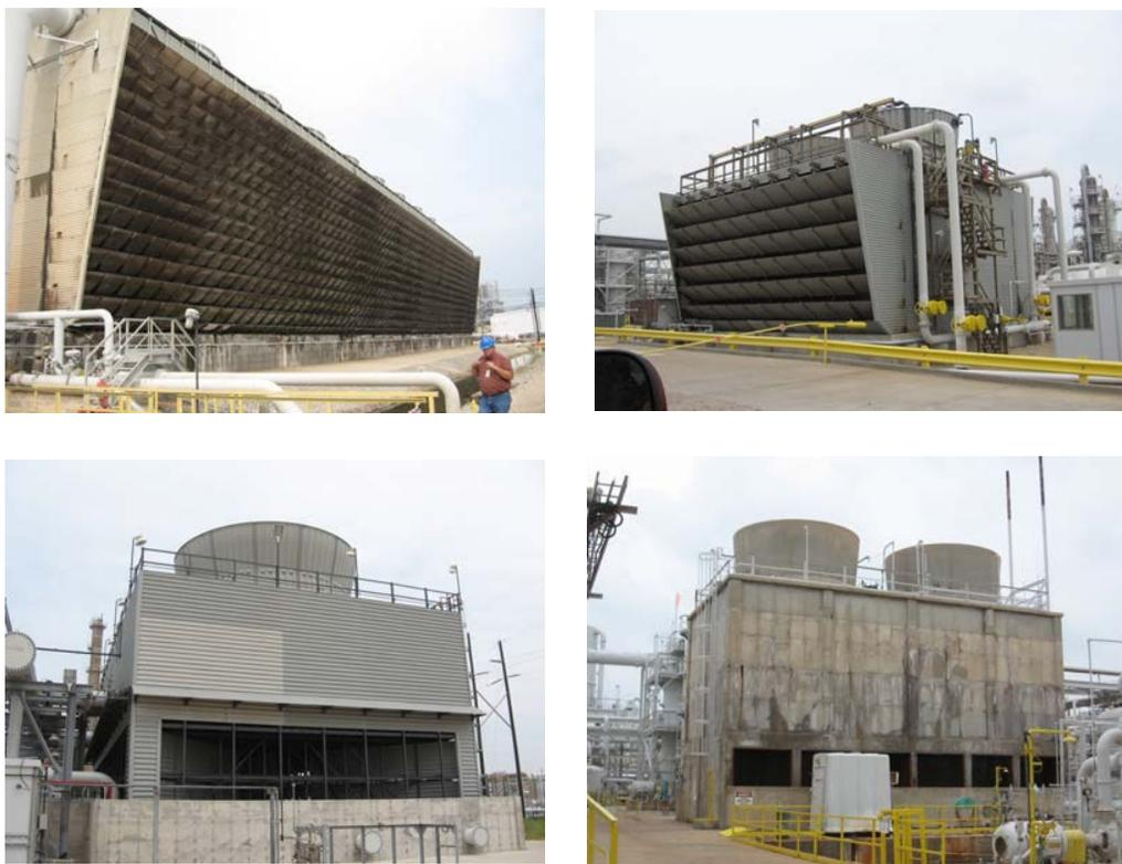
**Figure 92. Examples of Cooling Towers (Top Left: 9-Cell Wooden Tower; Top Right: 2-Cell Wooden Tower; Bottom Left: 2-Cell Concrete Tower; Bottom Right: 2-Cell Fiber-Reinforced Plastic Tower)**
