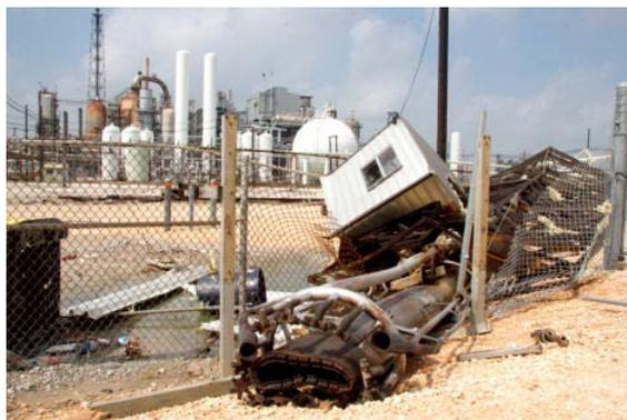
**Figure 97. Damage to a flare tower**
