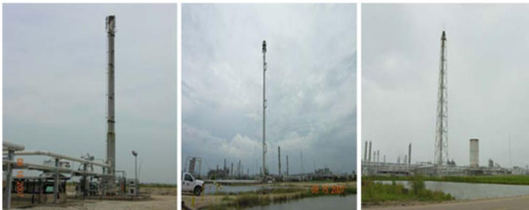
**Figure 96. Examples of flare towers (left: freestanding flare, middle: guyed flare, and right: derrick-supported flare)**
