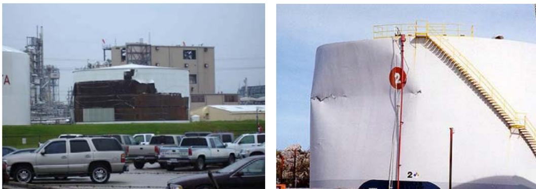
**Figure 88. Observed Wind Damage to Storage Tanks**
