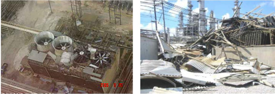
**Figure 93. Observed Hurricane Damage to Cooling Towers**
