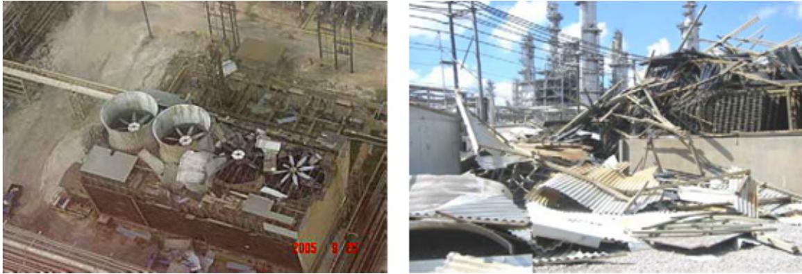
**Figure 95. Observed Hurricane Damage to Cooling Towers**
