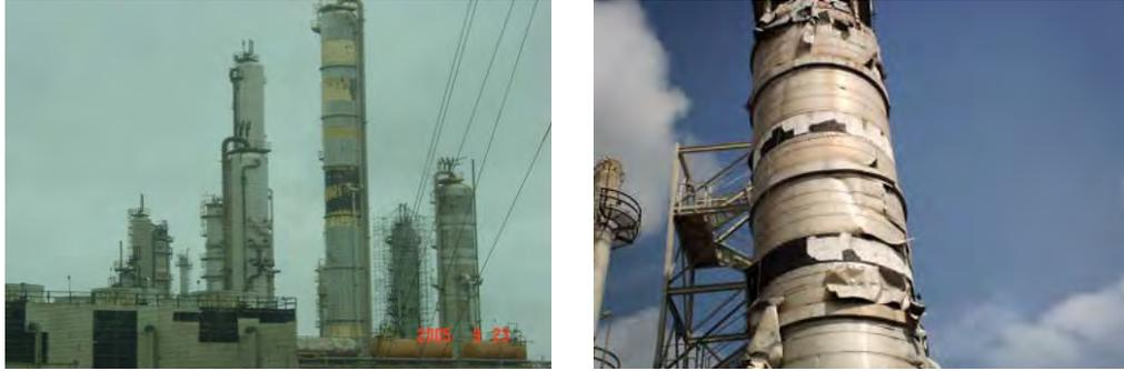
**Figure 87. Observed Hurricane Damage to Process Towers**
