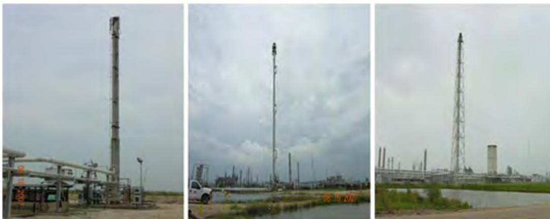
**Figure 88. Examples of Flare Towers (Left: Freestanding Flare, Middle: Guyed Flare, and Right: Derrick-Supported Flare)**
