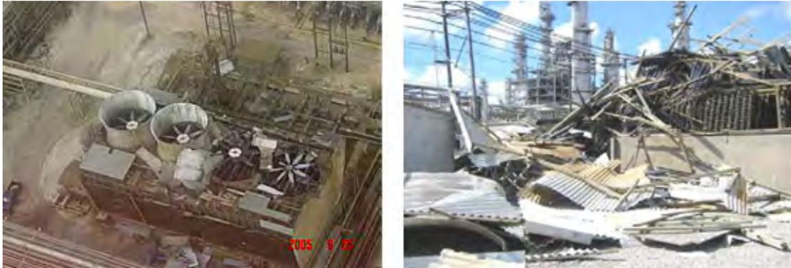
**Figure 85. Observed Hurricane Damage to Cooling Towers**
