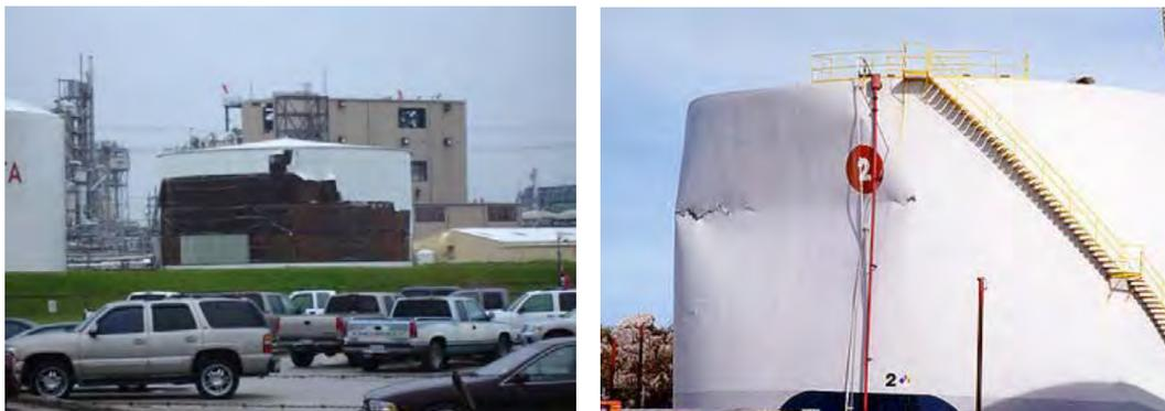
**Figure 80. Observed Wind Damage to Storage Tanks**
