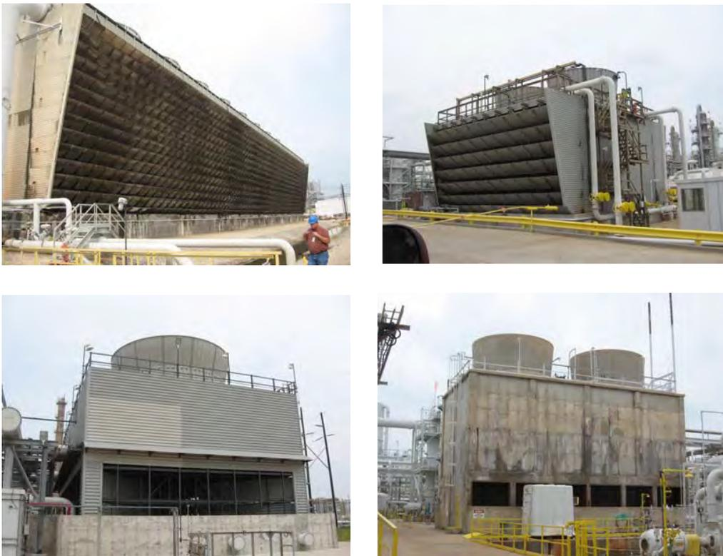
**Figure 84. Examples of Cooling Towers (Top Left: 9-Cell Wooden Tower; Top Right: 2-Cell Wooden Tower; Bottom Left: 2-Cell Concrete Tower; Bottom Right: 2-Cell Fiber-Reinforced Plastic Tower)**
