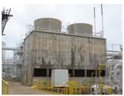
Figure 94. Examples of Cooling Towers (Top Left: 9-Cell Wooden Tower; Top Right: 2-Cell Wooden Tower; Bottom Left: 2-Cell Concrete Tower; Bottom Right: 2-Cell Fiber-Reinforced Plastic Tower)
