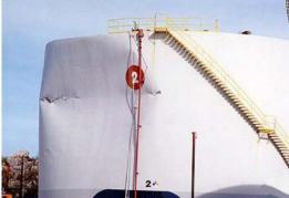
Figure 90. Observed Wind Damage to Storage Tanks
