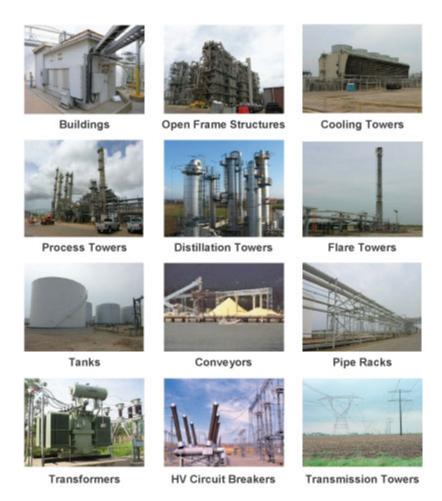
Figure 89. Examples of industrial facility components
