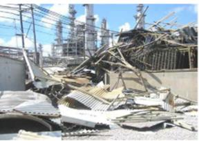
Figure 95. Observed Hurricane Damage to Cooling Towers
