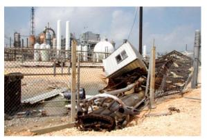
Figure 99. Damage to a flare tower
