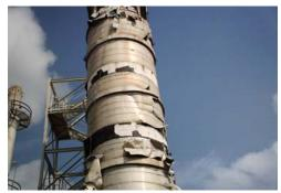
Figure 97. Observed Hurricane Damage to Process Towers
